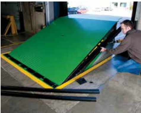
AFTER: ENERGY GUARD effectively seals off the perimeter gaps.
